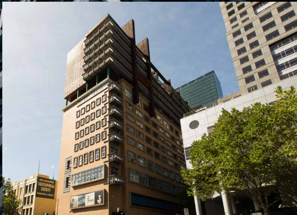
FIGURE 3 TRANSFORMATION OF TELSTRA EXCHANGE TO HERO APARTMENTS
